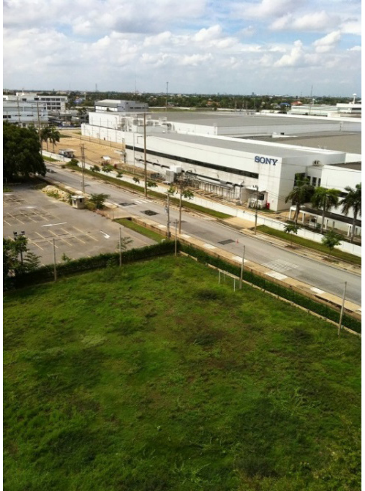
Factory that was damaged by the floods in 2011 and abandoned
