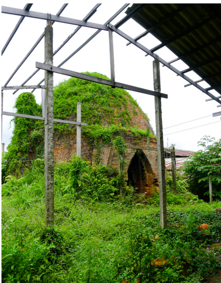
An oven used to bake bricks and terra cotta goods, products well-known in Vinh Long
